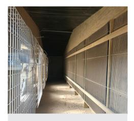
**D**. Light trap in a false wall in front of tunnel fans.
