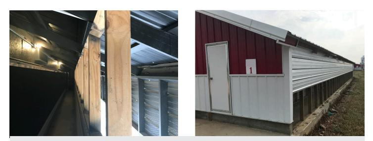
When using evaporative pads, a shaded inlet area (similar to the images shown above) can eliminate the need for inlet light traps. Alternatively, the best option would be to use a light trap with a considerably lower light reduction factor and pressure drop.
