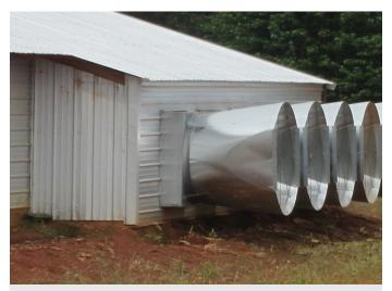
**E**. Tunnel fan light trap false wall installed in a vestibule plenum (dog house) in front of tunnel fans installed on the sides of the house.
