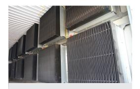
**B.** Light traps mounted over fans can reduce fan performance, and are not the best option in high-speed tunnel houses.
