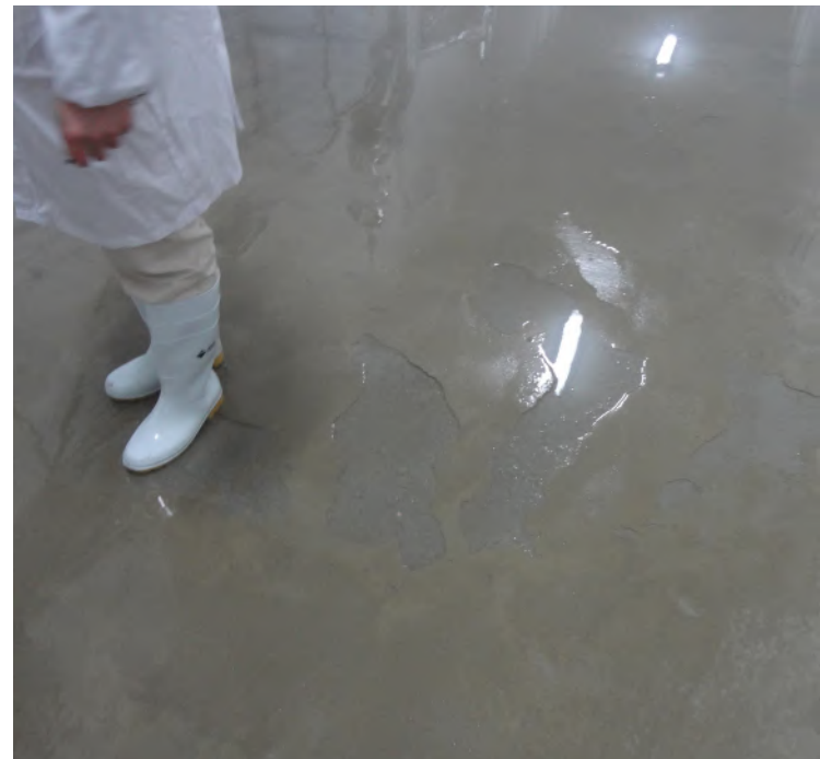
The facility floors should be designed to drain well, prevent standing water and free of cracks and holes. Here, cracks and chips in the floor hold water and prevent the floor from completely drying.
